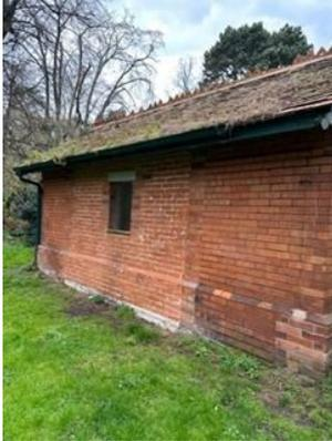
Pavilion pointing to brickwork where extension was removed needs attention. Specialist required to blend brick colours to match. Rubbish to be cleaned off roof. Any proposal to install security gates should be done in consultation with Howley Hayes Conservation Architects.
