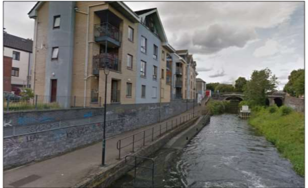
Existing Site Layout showing tow path, adjacent apartments & jetty.
