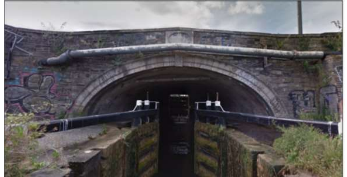
Existing Site Layout Showing Binns Bridge and 2 nd Lock
