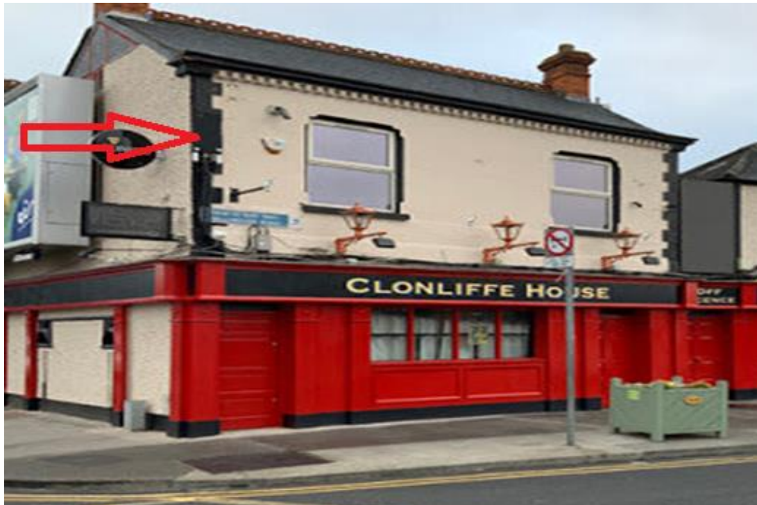
Clonliffe House: Antenna attached to the front of the building painted black to match the front of the building.
