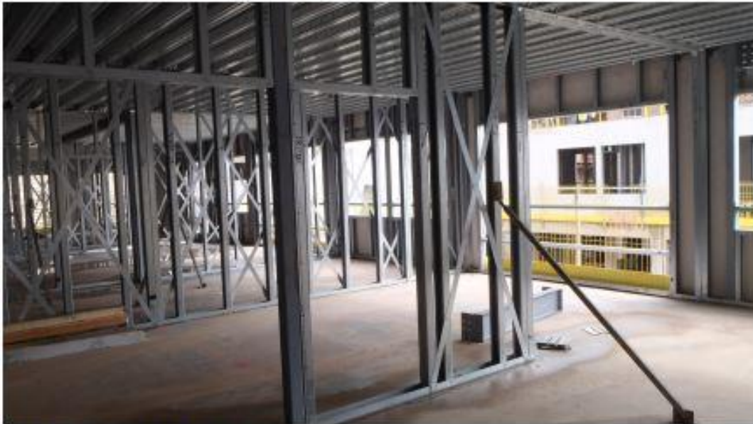
▲ Pre fabricated internal stud partitions
