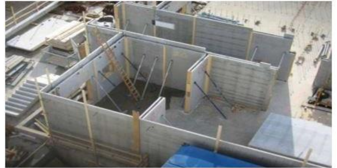
▲ Precast concrete structure
