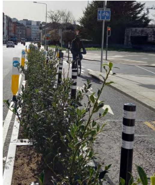
Planter protection on Parnell Square East Protected Contra-Flow Cycle Lane
