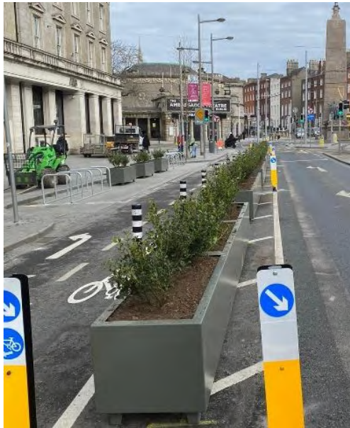
Planter protection on Parnell Square East Protected Contra-Flow Cycle Lane
