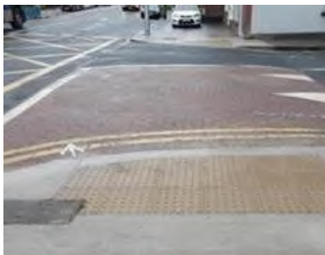
Tactile paving Monck Place / Phibsborough Road junction
