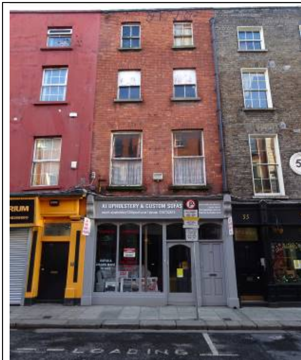
Fig.3: Principal/west elevation. Note the machine made red brick façade reflecting a re-facing of the early 18 th century building c.1900.
