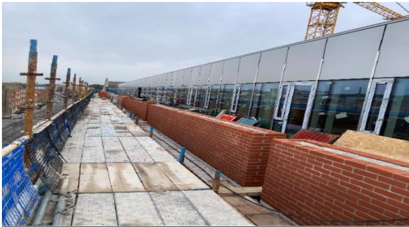
Works of the Façade 5 th Floor Dominic St. Elevation
