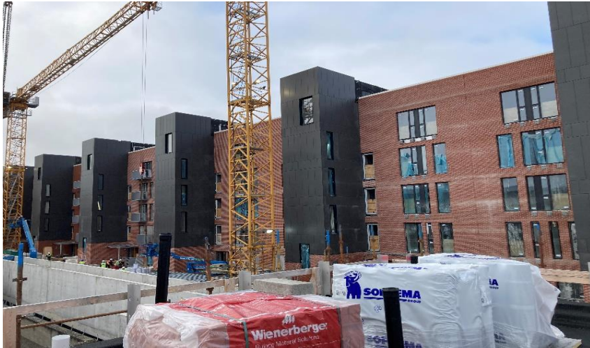
Rear Elevation of the Project
