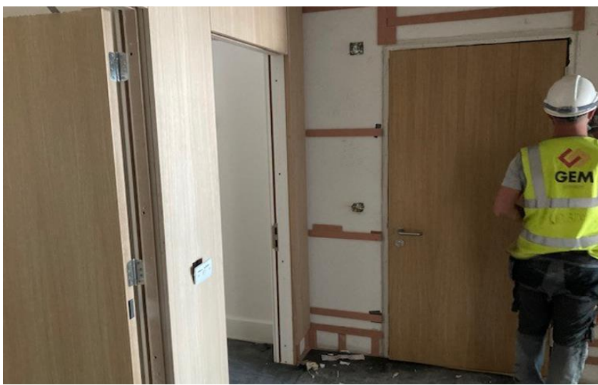
Wood Panelling Ongoing In Apartments
