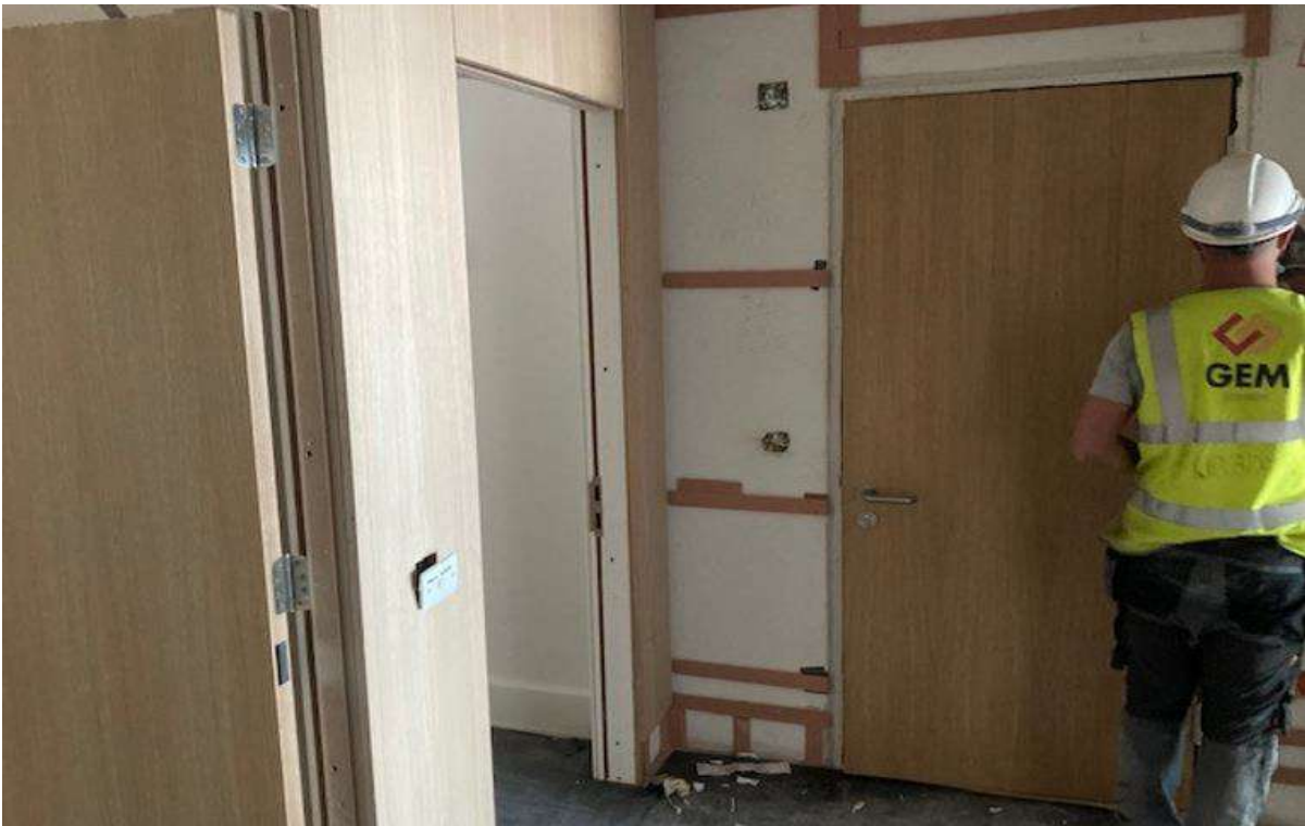
Wood Panelling Ongoing In Apartments
