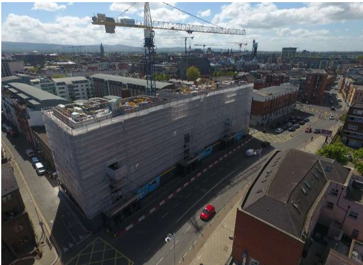
View of Site Works Progressing
