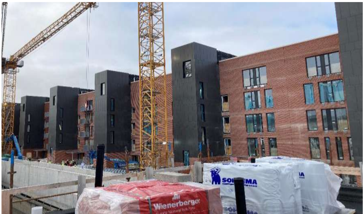
Rear Elevation of the Project
