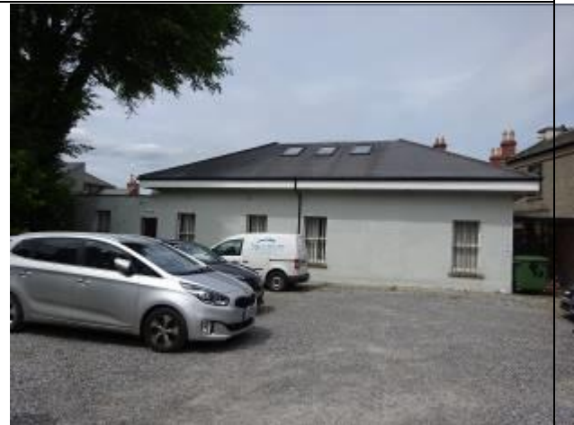
Fig.6: Aspect of 19 th century single-storey annexe with replacement roof (c. 2002) within the curtilage of Garland House and not proposed for protected structure status. .
