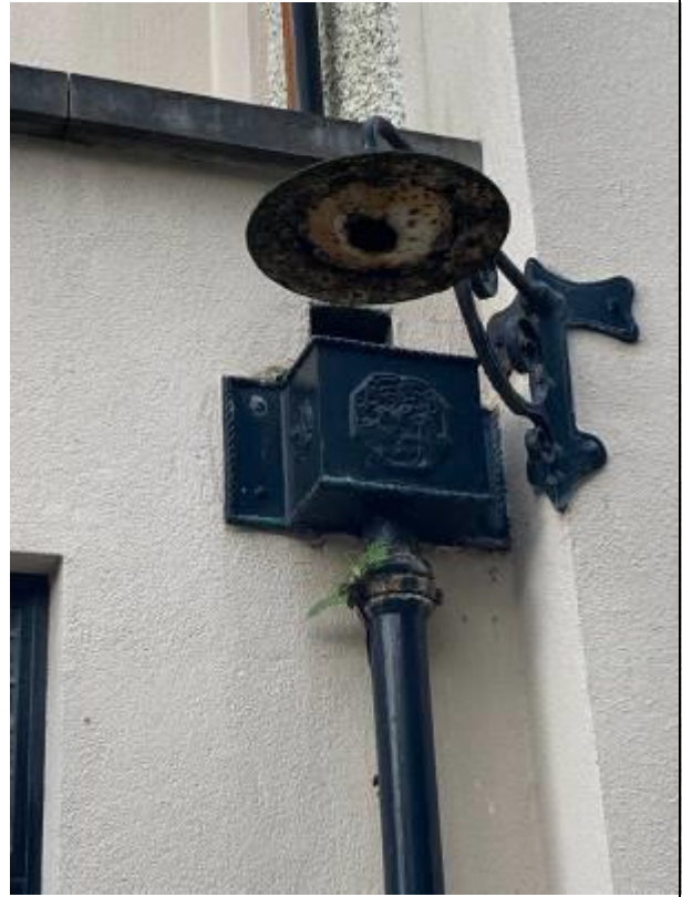
Fig.8: Cast-iron box hopper and early electric lighting sconce.
