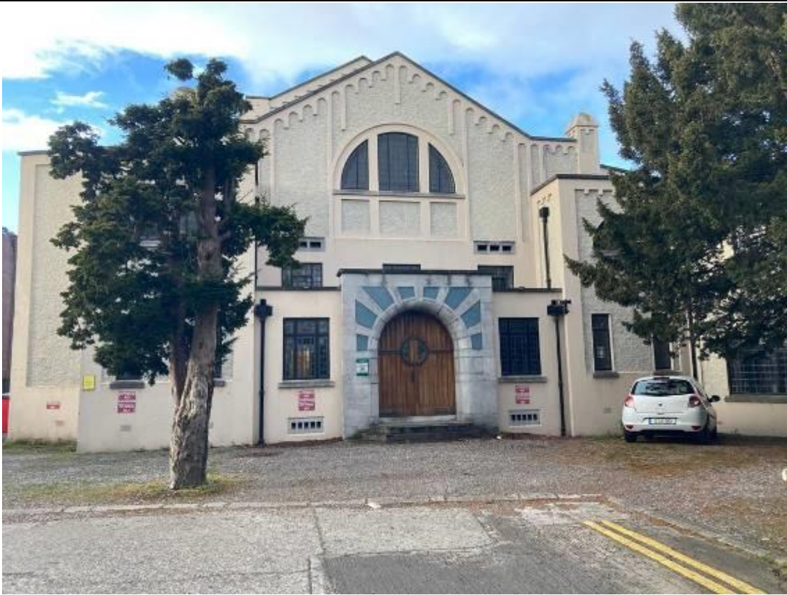
Fig.4: Principal/south elevation of Garland House (former Second Church of Christ Scientist). Note the yew tree to the front site which appears on early archival images dating to c.1929.
