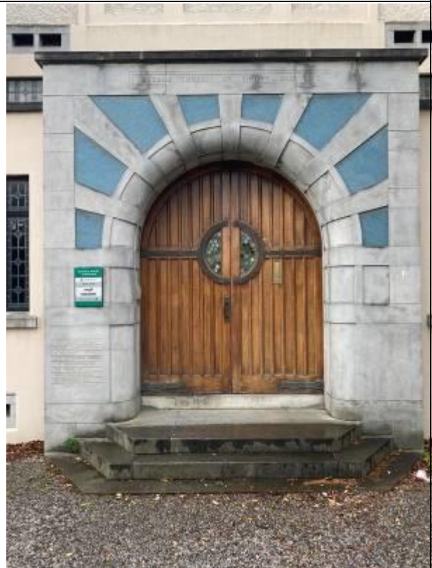
Fig.10: Stradbally limestone door surround incorporating mosaic sunburst detailing.
