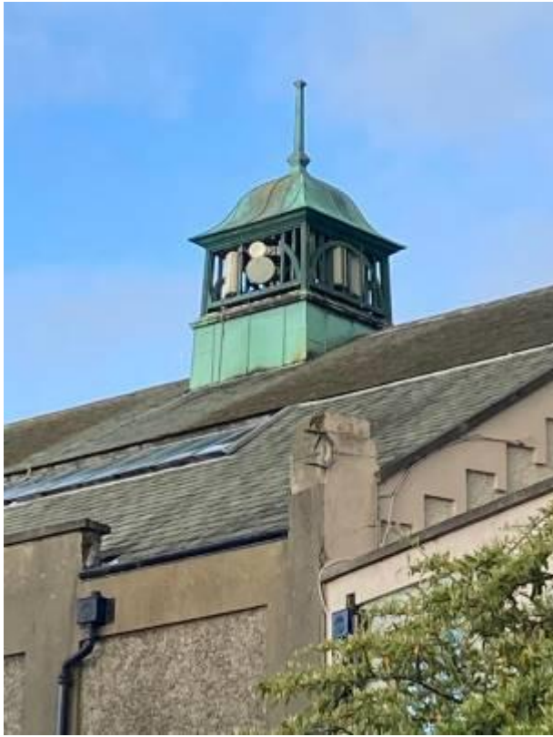
Fig.7: Ventilator/lantern to roof of auditorium. Note the Westmoreland slate roof and in-line band of rooflights mid-pitch.
