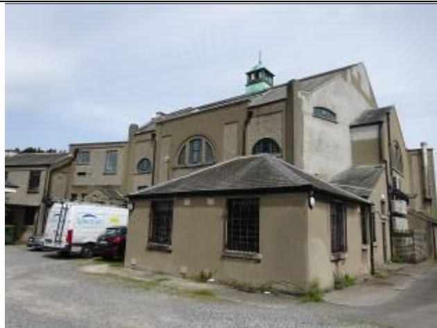
Fig.5: Aspect of Garland House (former Second Church Christ Scientist) taken from the southwest.
