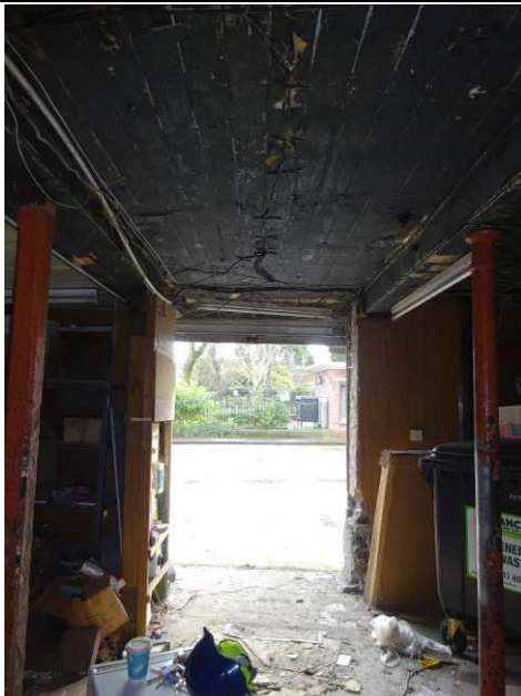
Fig.11: Main shop entrance flanked by cast and timber support pillars and timber beams above
