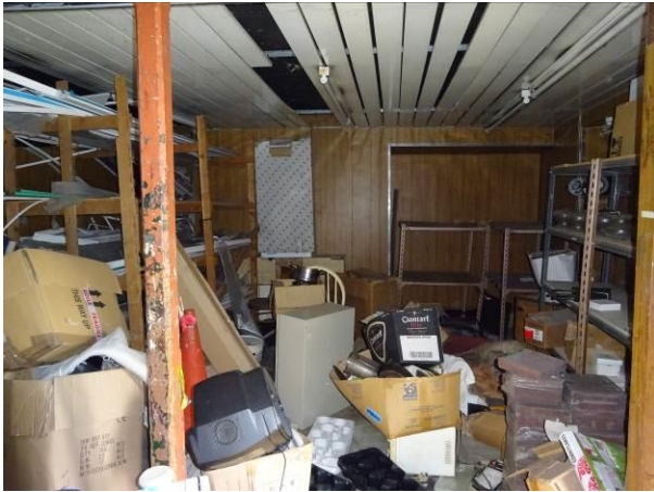
Fig.9: Open plan shop looking north with chamfered post supporting first floor internal walls and chimney stack in north wall
