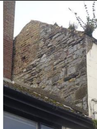
Fig.8: Rubble stone gable end to south with brick coursing to eaves and traces of an original brick chimney stack
