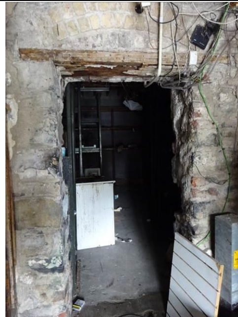
Fig.12: Rear door opening directly opposite main entrance lime washed with brick arch and remains of lath and plaster to timber lintel
