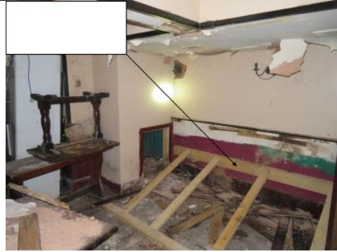
Figure 2 - Temporary supports applied to basement level external walls.
