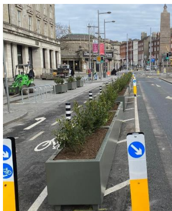
Planter protection being installed on Parnell Square East Protected Contra-Flow Cycle Lane
