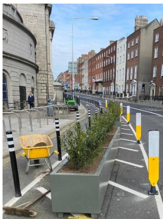
Planter protection being installed on Parnell Square East Protected Contra-Flow Cycle Lane
