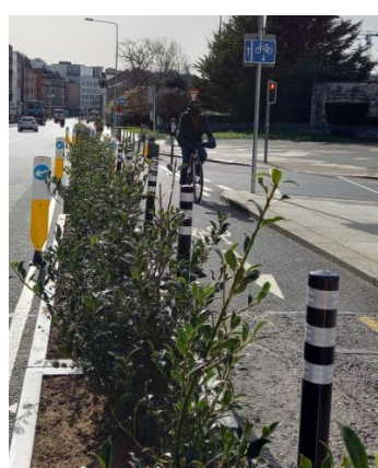
Planter protection being installed on Parnell Square East Protected Contra-Flow Cycle Lane
