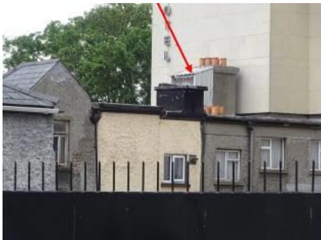
Fig.6: Rear aspect of No.8 showing significant chimney stack (arrowed) indicative of an early date.
