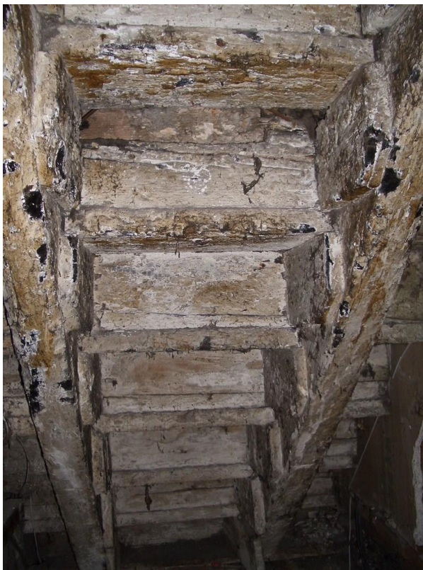
Underside of stairs to basement with remains of distemper (whitewash)
