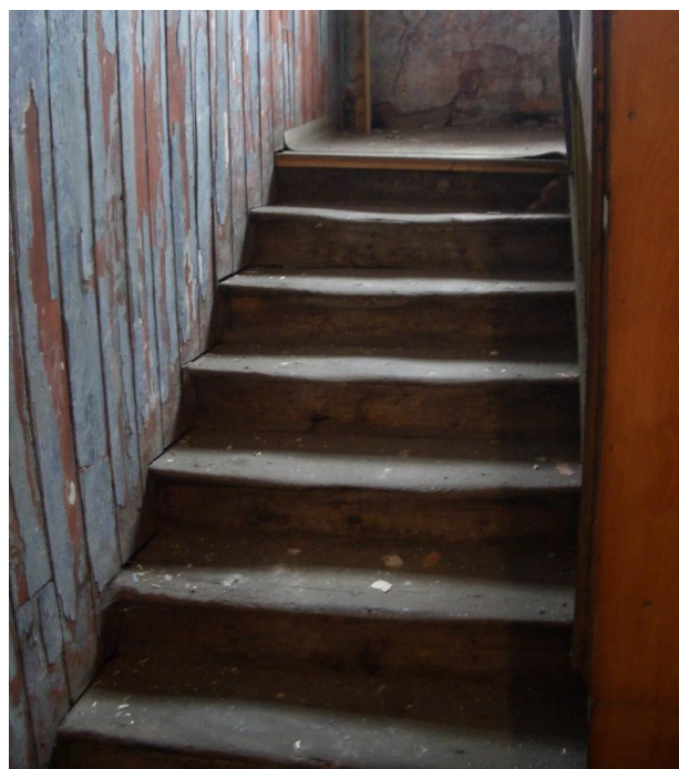
Stairs from 2 nd to 3 rd floor, looking to half landing showing early plank partition
