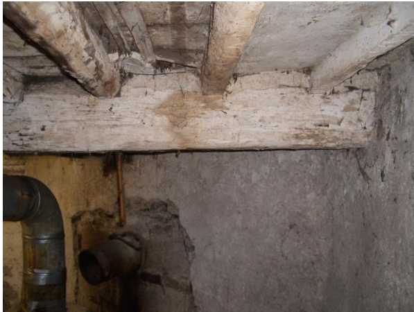
Rear basement bressumer, looking to chimney. Note plaster sarking between joists.
