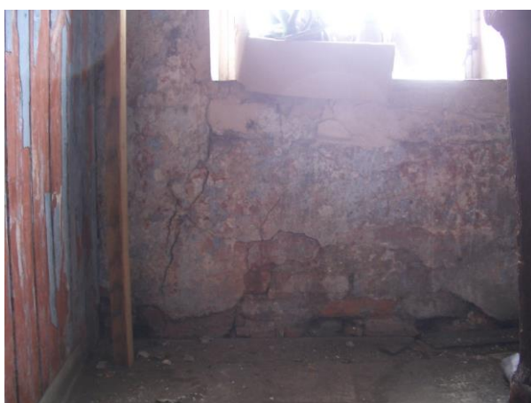
East window spandrel, third floor. Early plank partition also visible.
