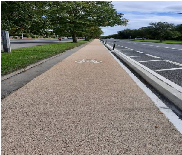
Extruded kerb on cycle lane on Griffith Avenue
