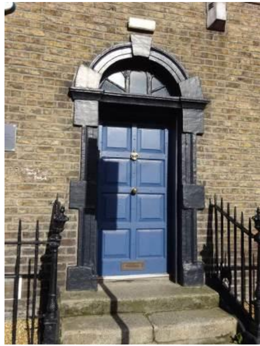
Fig. 7: Block-and-start doorcase to front elevation.
