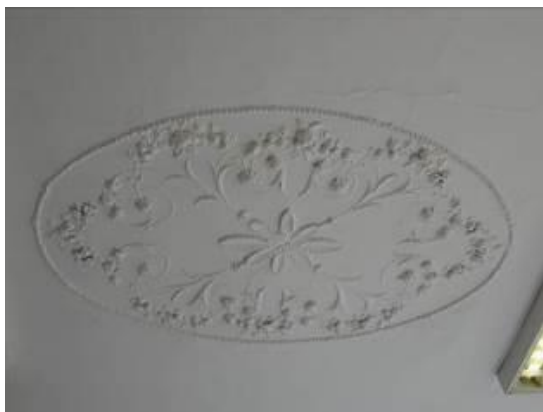
Fig. 8: Ceiling rose to ground floor, east room.
