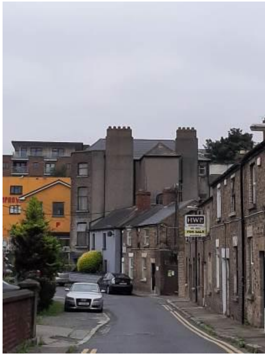
Fig. 6: Site context from north showing two-storey early twentieth houses to Kearns Place
