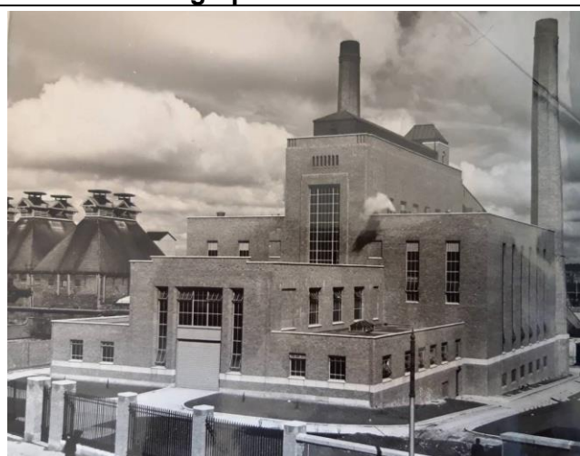
Power House, St James's Gate Brewery, Dublin 1946-9 (Copyright – A. Guinness Son & Co. Ltd.; Image sourced in Irish Architectural Archive). This image, taken shortly after the building's completion, shows the copper roofs to the upper sections and the coal conveyor to the rear of the Boiler House.
