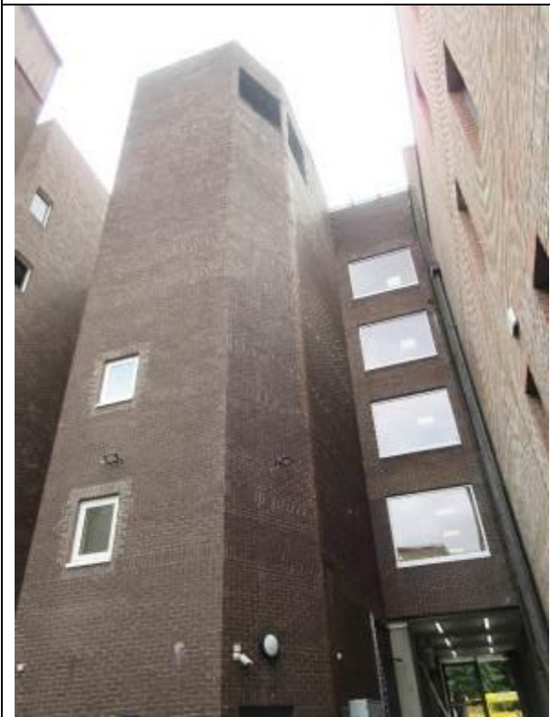
Service block and west bay to rear elevation
