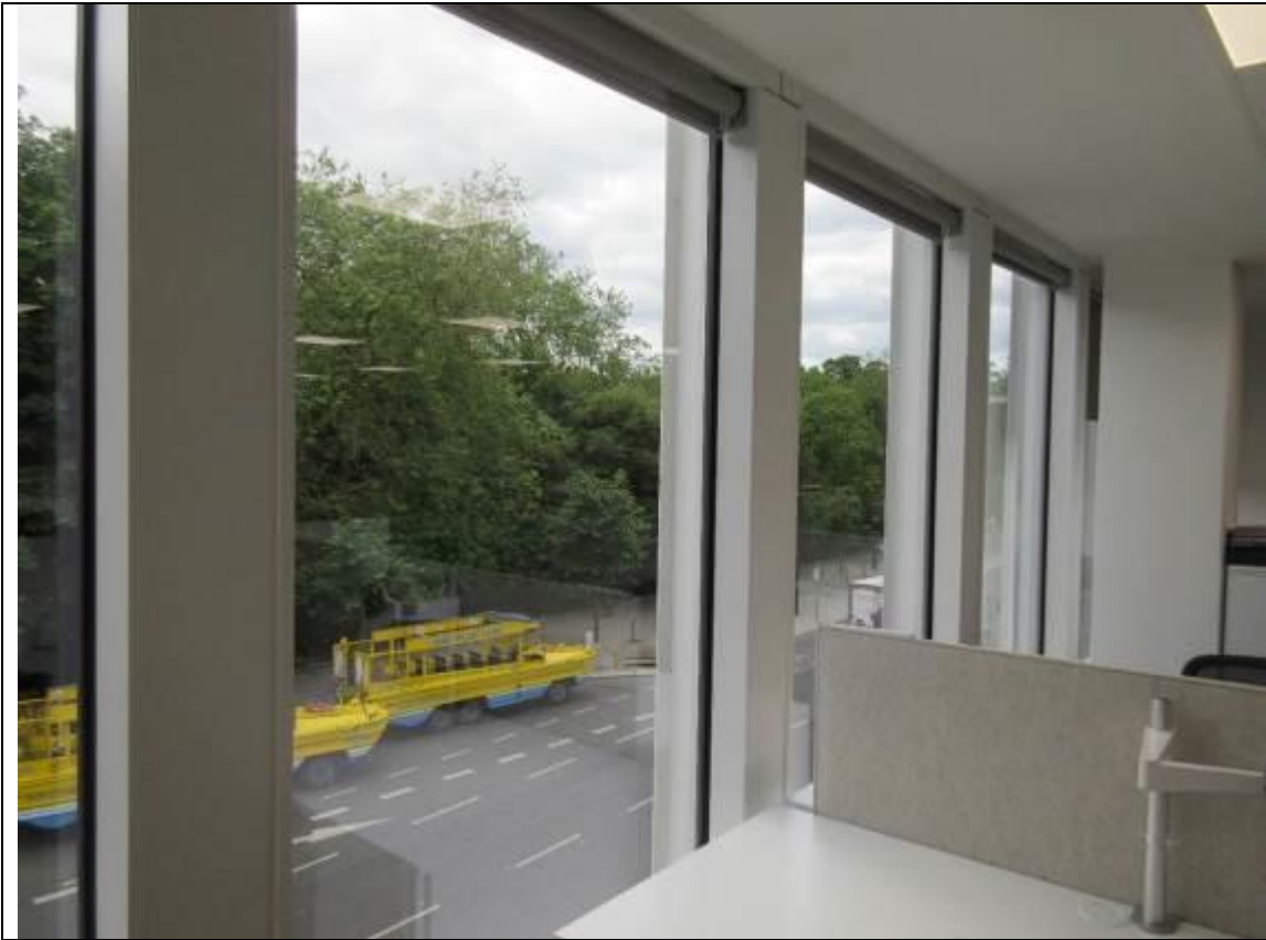
Façade, detail, second floor
