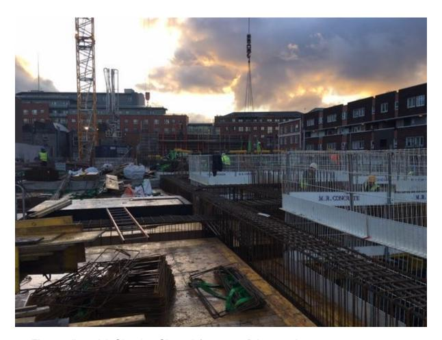
1st Floor podium slab GL 13b - GL 5 reinforcement fixing ongoing.
