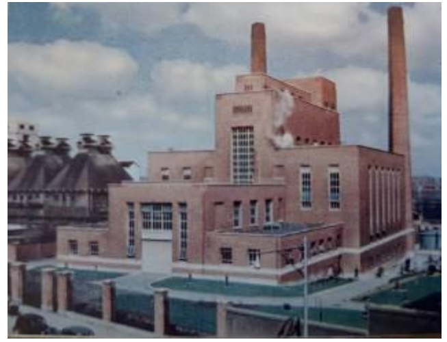
Image of Power Station dated 1959 from The Guinness Harp Bicentenary Issue 1759-1959 ; note the coal conveyor and copper roofs have been removed and the structure above the Boiler House is no longer clad in copper.
