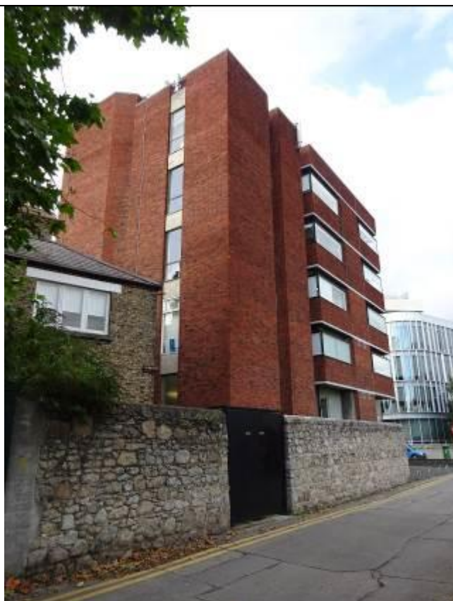
10 Burlington Road, Dublin 4, west elevation and rear boundary wall
