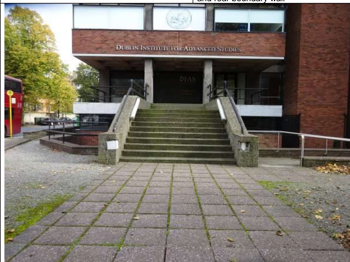
10 Burlington Road, Dublin 4, entrance
