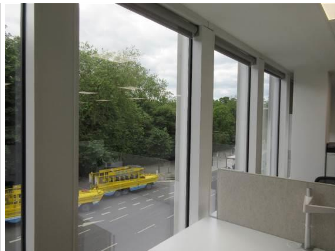
Façade, detail, second floor
