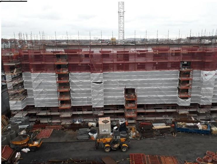
Cluid have advised that “The project continues to progress well.” The raising of the external walls continues with the second floor extension nearing completion on two of the four blocks.
