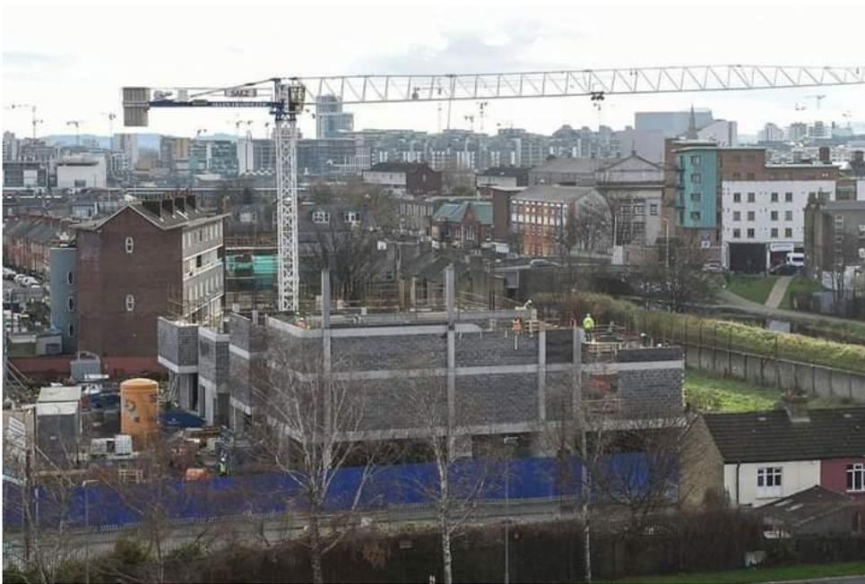
Foundation works of new Handball alley are now complete. Ground and first floor brick work has near completion with second floor beginning. Construction on the new Croke Villas Apartments will commence once the Handball Alley is completed.
