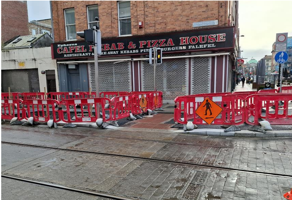
Figure 6 New buildout Capel St/Abbey St junction Feb 2025 under construction
