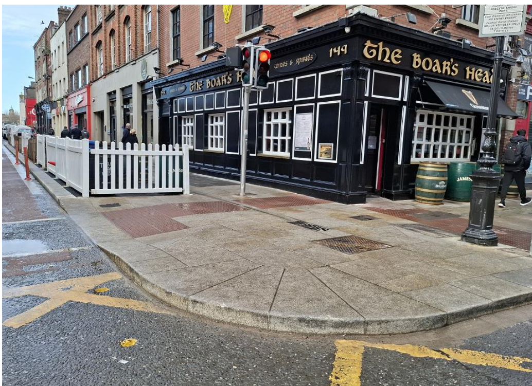
Figure 5 Capel St/Abbey St junction Feb 2025 with new buildout
