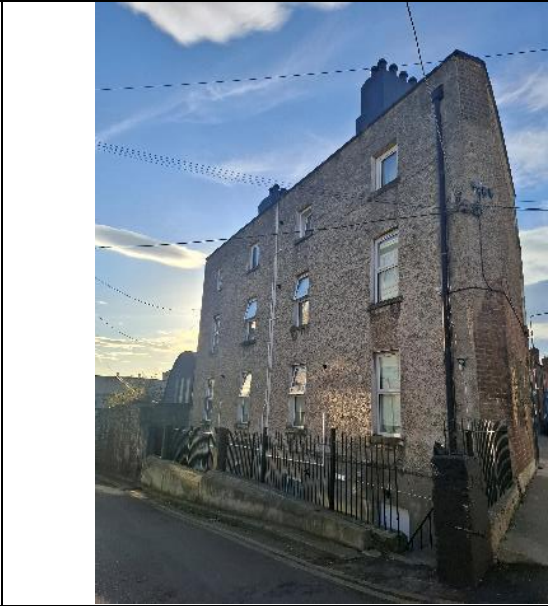
Fig. 4: East elevation from northeast
