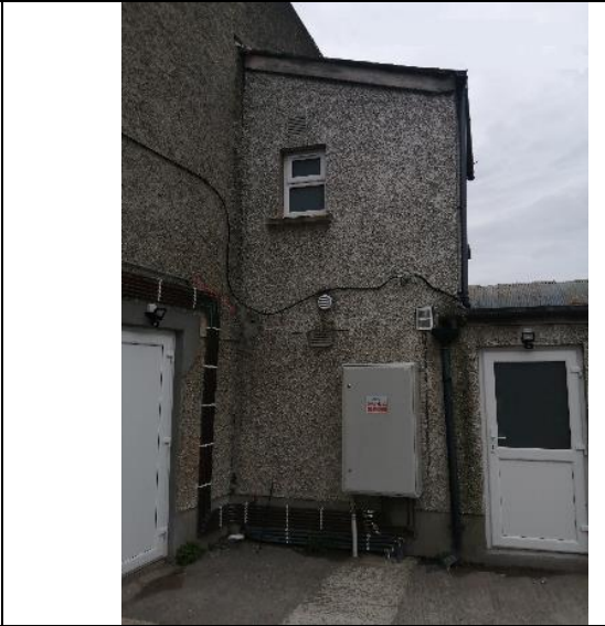
Fig. 6: Two-storey extension to west
