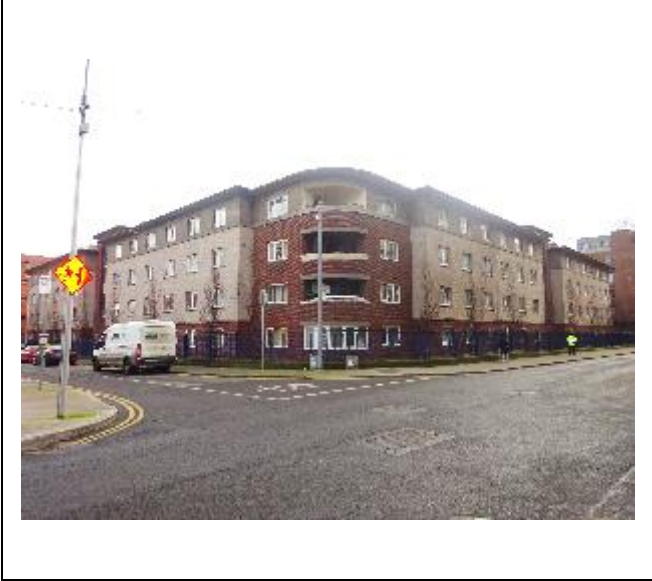
Fig. 4: View from northwest
