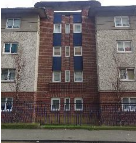
Fig. 8: Central recessed bays to west elevation
