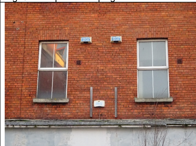
Fig. 10: First floor windows.
