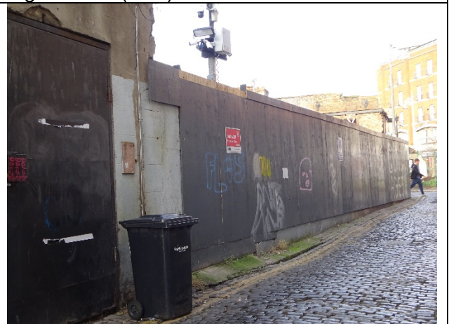
Fig. 7: Rear boundary to Jervis Lane Upper.
