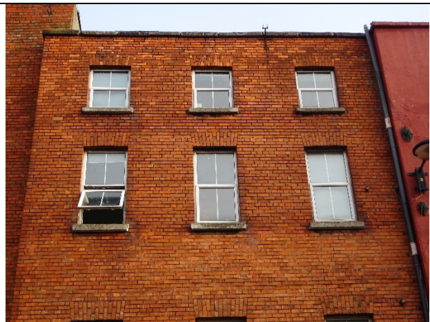
Fig. 9: Windows to second and third floors.
