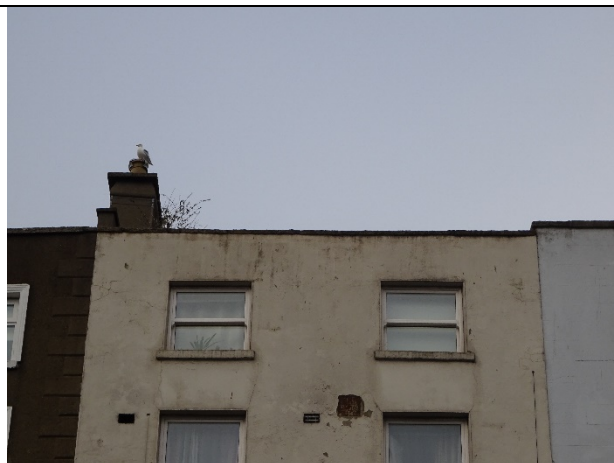
Fig. 9: Third floor windows.
