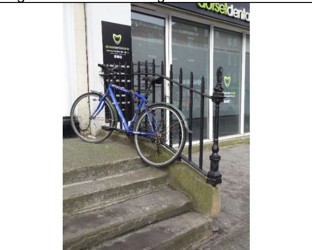
Fig. 13: Railings to entrance steps.
