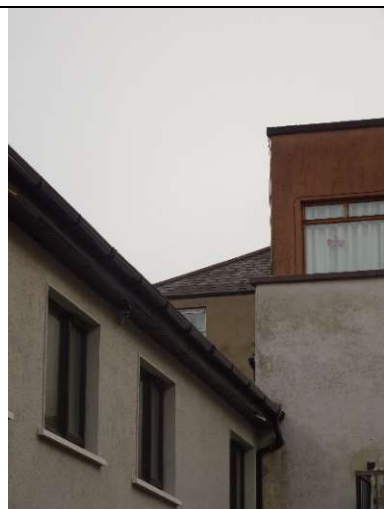
Fig. 6: Rear elevation, visible over buildings to Blessington Court.
