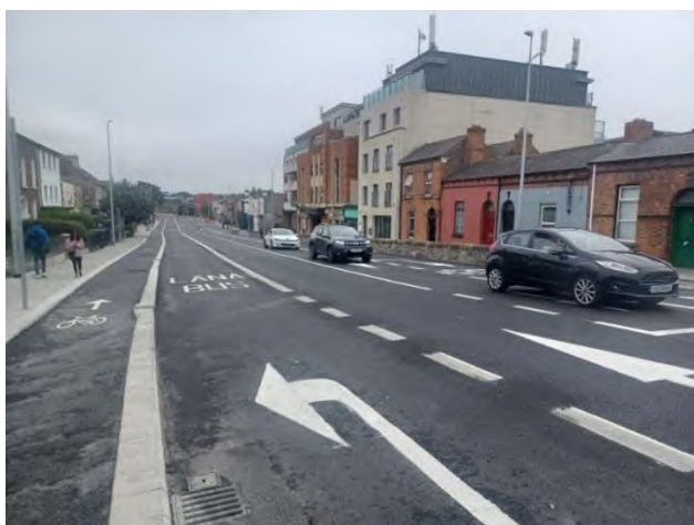
C2CC – North Strand Road Diversion Removed for inbound traffic
