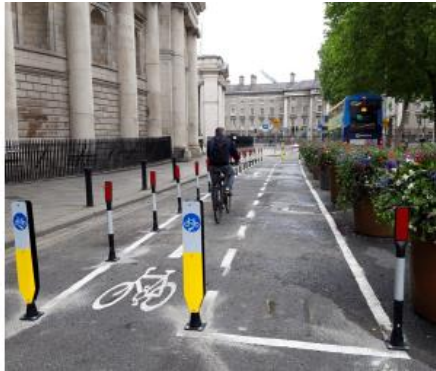
New protected cycle lane in Dame Street, Dublin City Centre
