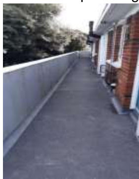
New anti-slip landing
