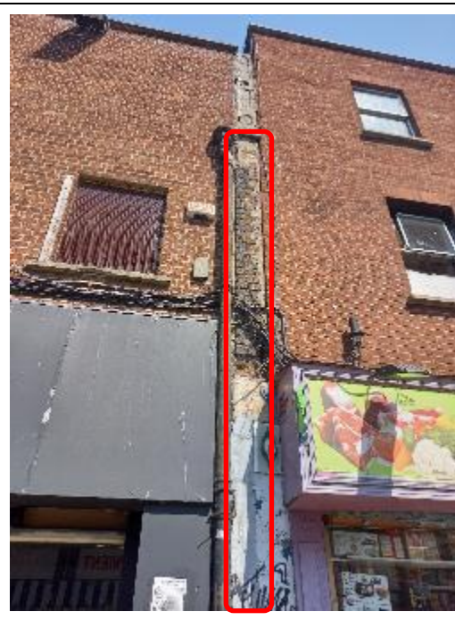
Fig. 4: Historic party wall between 12 and 13 Moore Street; outlined in red
