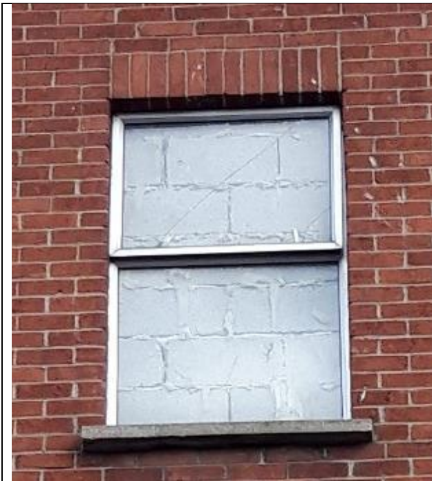
Fig. 5: First floor window opening with modern frame
