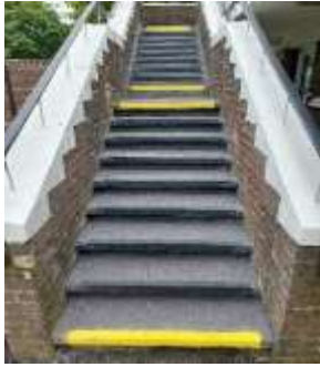
New anti-slip stairs.
