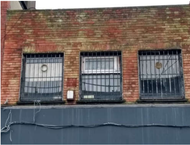
Fig. 2: 19 Moore Street with fixed pane and top opening window.
