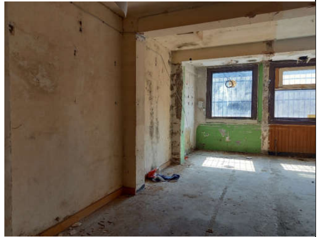
Fig. 3: 19 Moore Street, view of first floor.
