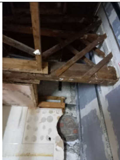
Figs. 4 & 5: View of Belfast Truss supporting curved roof.
