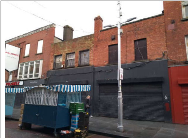
Fig. 2: View of 18 Moore Street (RHS) with 19 Moore Street (LHS)
