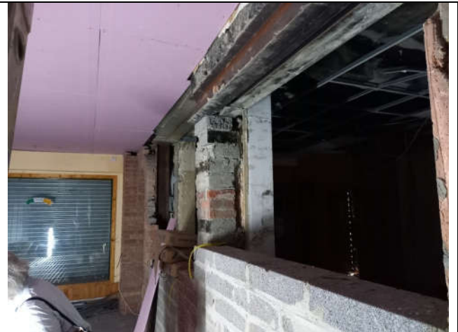
Fig. 3: ground floor interior of 18 Moore Street
