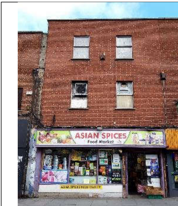
Fig. 3: West elevation of 12 Moore Street
