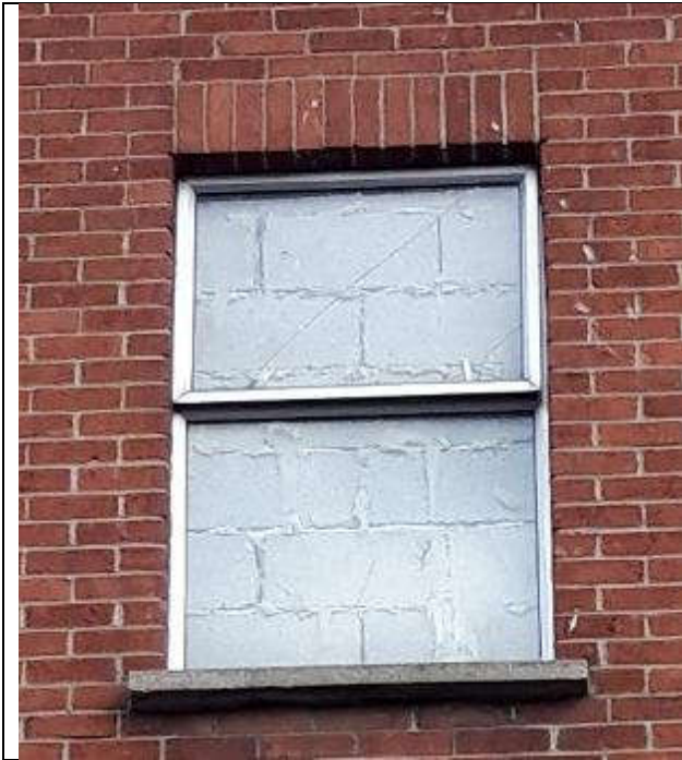
Fig. 5: First floor window opening with modern frame
