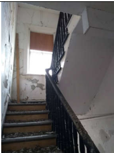
Figure 5: Surviving dogleg, open string staircase with continuous handrail.
