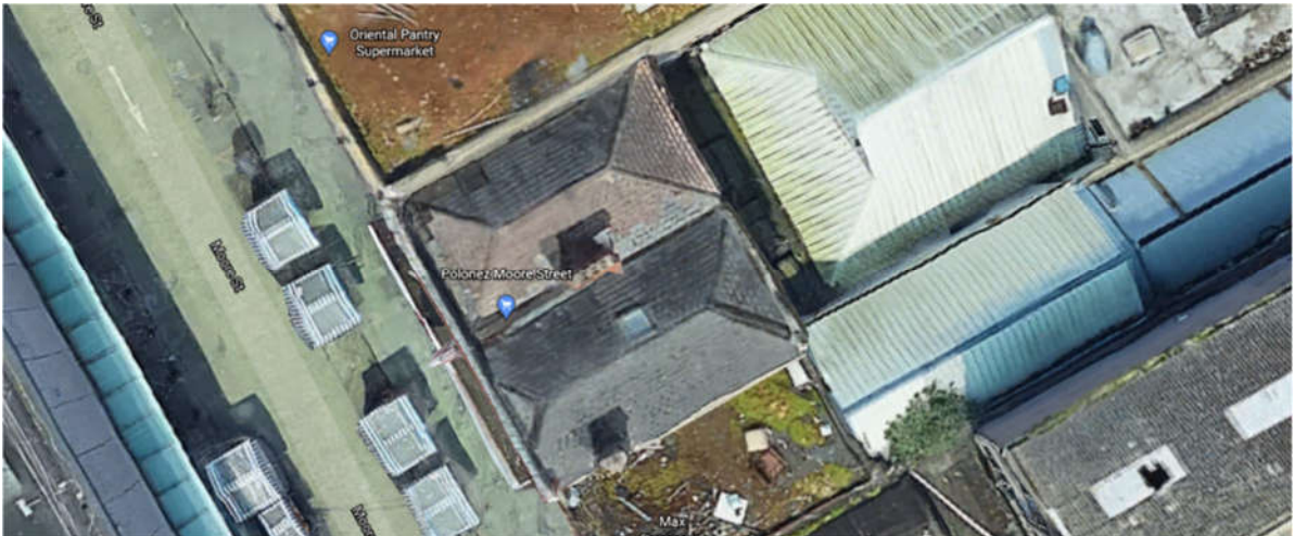
Fig. 7: 20/21 Moore Street showing early roof form perpendicular to street with hipped sections to front and rear (Google Earth 04/12/20)
