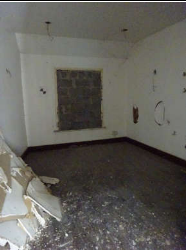
Fig. 7: Second Floor front room with timber floor boards and blocked up window opening
