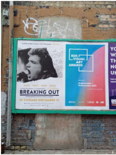
Fig. 5: Blocked up side door to Henry Place.
