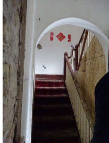
Fig. 6: Staircase viewed from first floor
