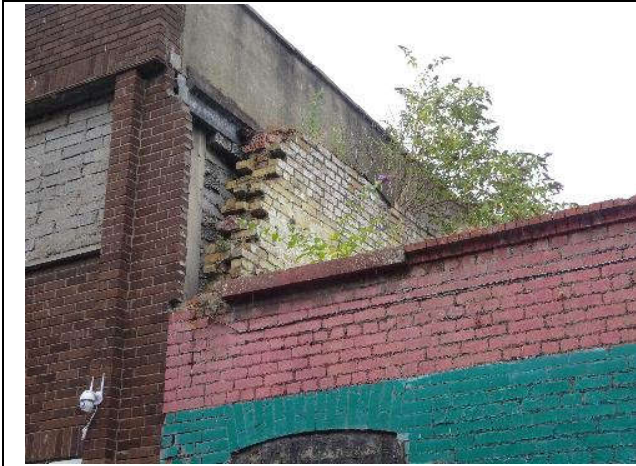
Fig. 5: 17/18 Henry Place, upper section of western party wall to 16 Henry Place.
