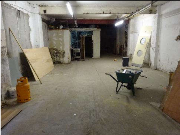
Fig. 7: Interior view of ground floor looking south.
