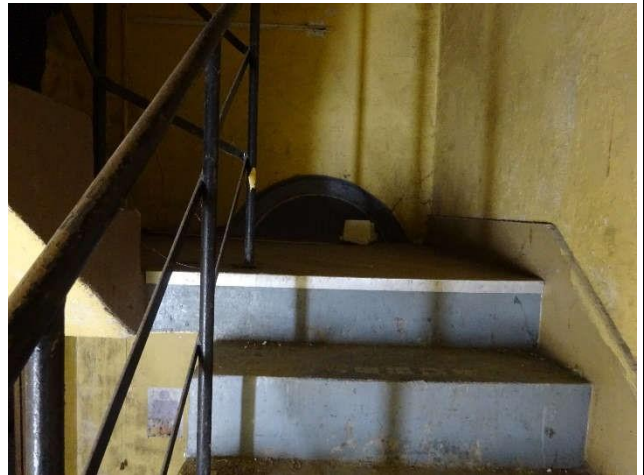
Fig. 6: Concrete stairs with fanlight from blocked door opening visible
