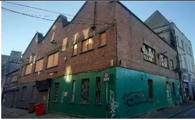
Fig. 3: Nos. 4-8 Henry Place - view from northeast
