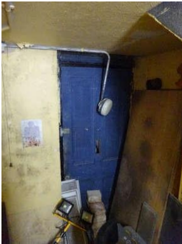
Fig. 5: Historic door opening to east elevation, now blocked
