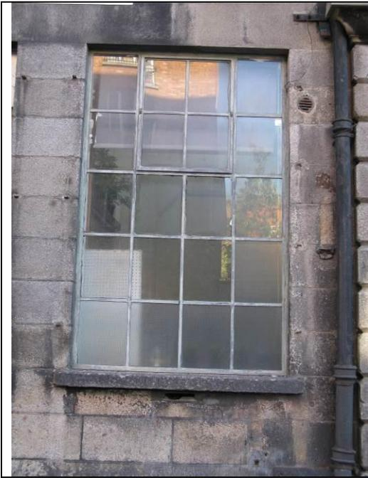
Fig. 7 Early metal window with central pivot opening section on Loftus Lane
