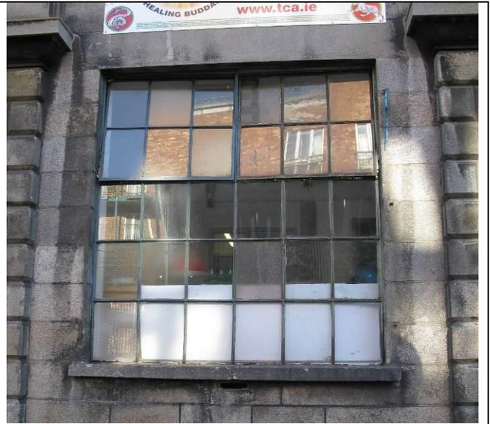
Fig. 8 Original metal window with pair of central pivot opening sections retaining panes of early glazing on Kings Inn Street elevation
