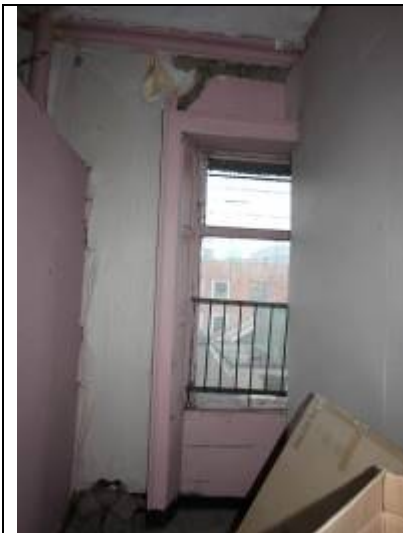
Fig. 9 Surviving window joinery and cornice to rear wall at first floor; note partition cutting open
