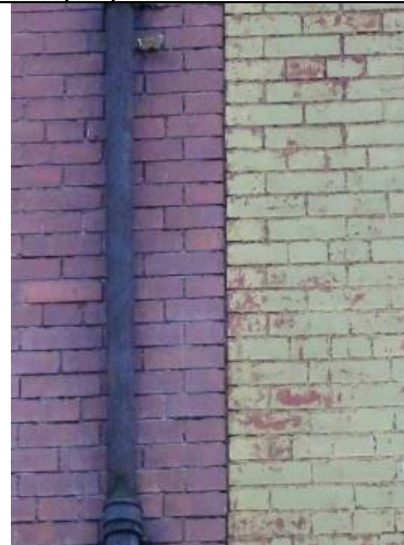
Fig. 6 Break in brickwork between Nos.46a and 46
