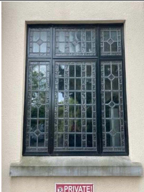
Fig.9: Painted steel frame and leaded light window with limestone cill.
