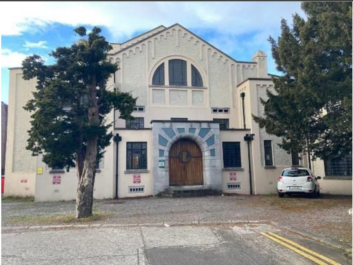
Fig.4: Principal/south elevation of Garland House (former Second Church of Christ Scientist). Note the yew tree to the front site which appears on early archival images dating to c.1929.
