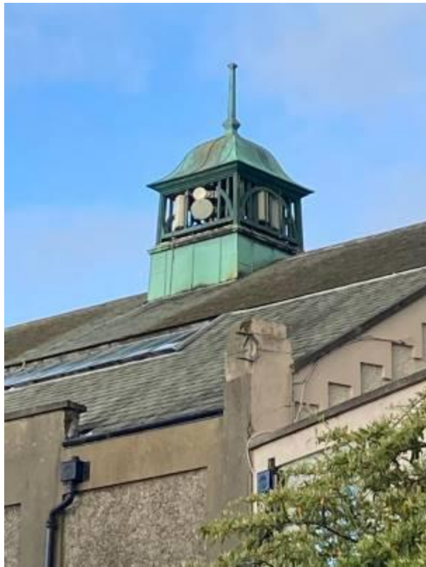
Fig.7: Ventilator/lantern to roof of auditorium. Note the Westmoreland slate roof and in-line band of rooflights mid-pitch.
