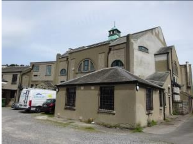
Fig.5: Aspect of Garland House (former Second Church Christ Scientist) taken from the southwest.
