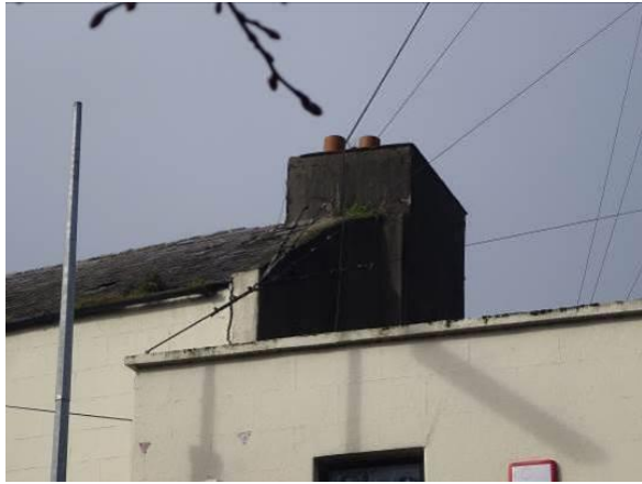
Fig.7: Huge corner chimney stack shared with No. 148
