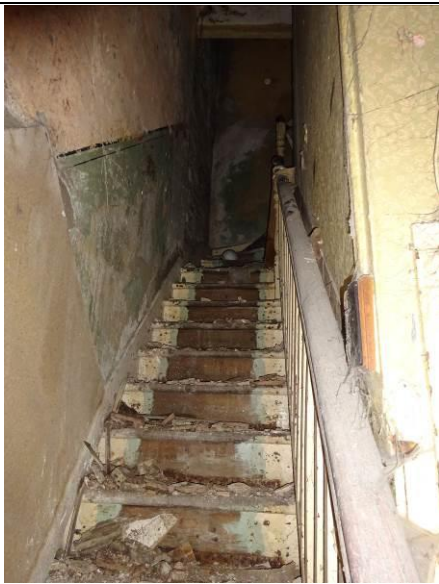
Fig.15: Timber staircase running up back wall with lime plastered walls with historic paint finish
