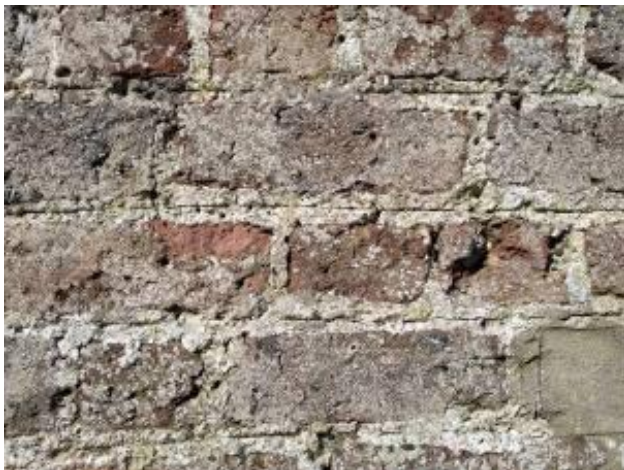
Note surviving penny struck lime mortar joint.
