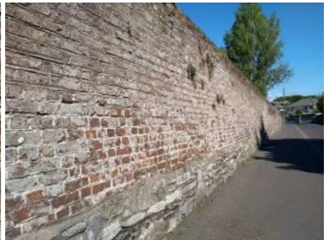
Note surviving penny struck lime mortar joint.
