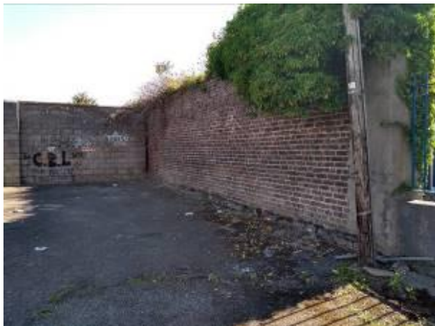
Former walled garden wall. Brick on western side and calp limestone on eastern side.
