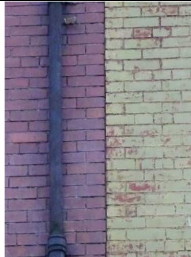
Fig 6: Break in brickwork between Nos.46a and 46
