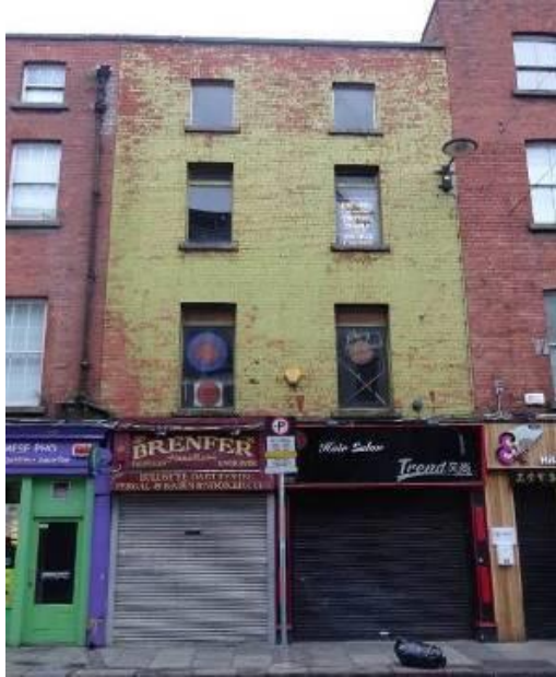
Fig 3: Front (east) elevation 46 (left) and 45a (right)
