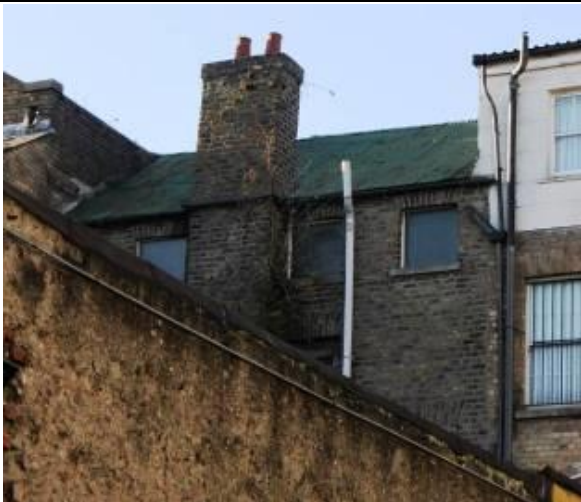
Fig 5: Rear elevation from northeast
