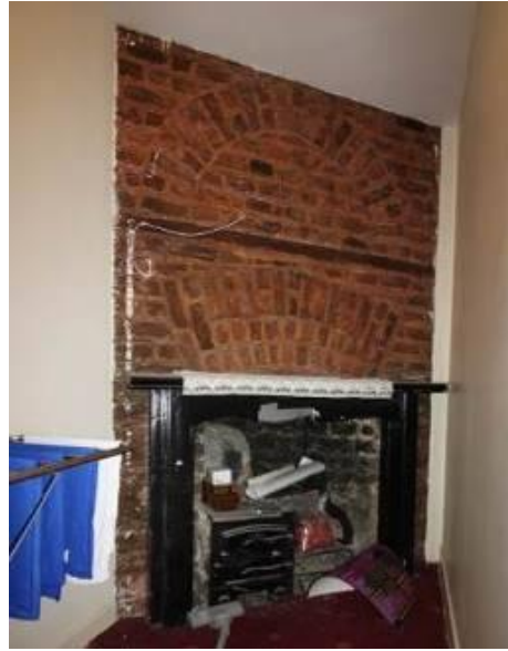
Fig 10: Corner fireplace to south party wall, No.45a
