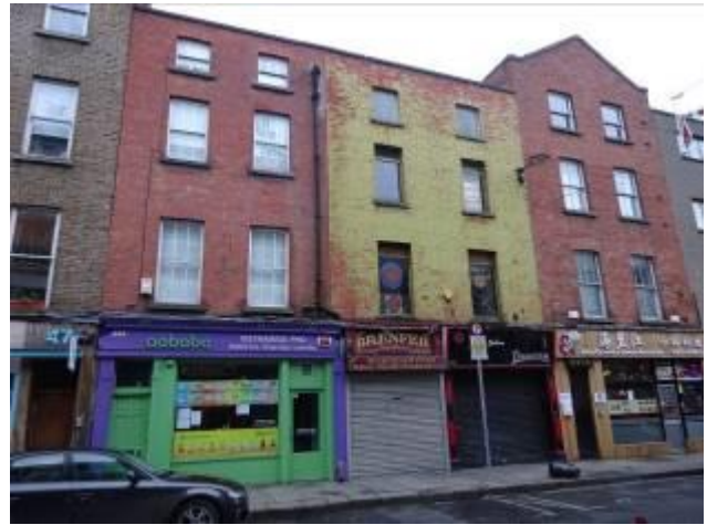
Fig 4: Nos. 46a and 46/45a from east; note shared downpipe between the two properties
