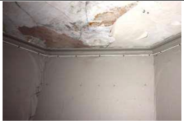
Fig 16: Historic cornice to second floor, angled around corner fireplace
