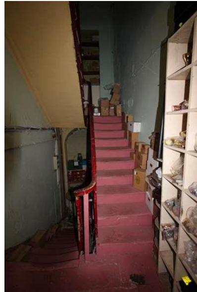
Fig 12: View of stairs
