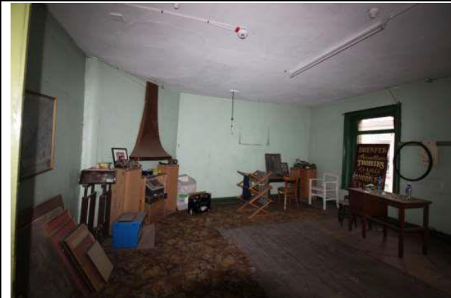
Fig 15: Second floor room looking southwest with corner fireplace and surviving historic window joinery
