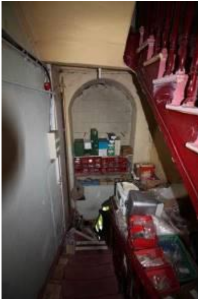
Fig 11: Stairs from ground to first floor with blocked round-headed opening
