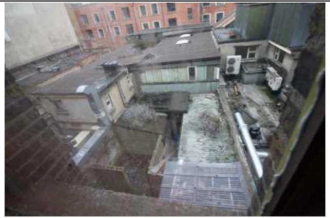
Fig 18: View of rear yard from second floor
