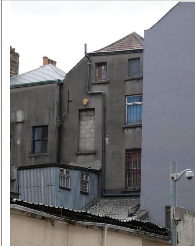
Fig. 5: Rear elevation from northeast showing part gabled elevation and half-hipped roof.
