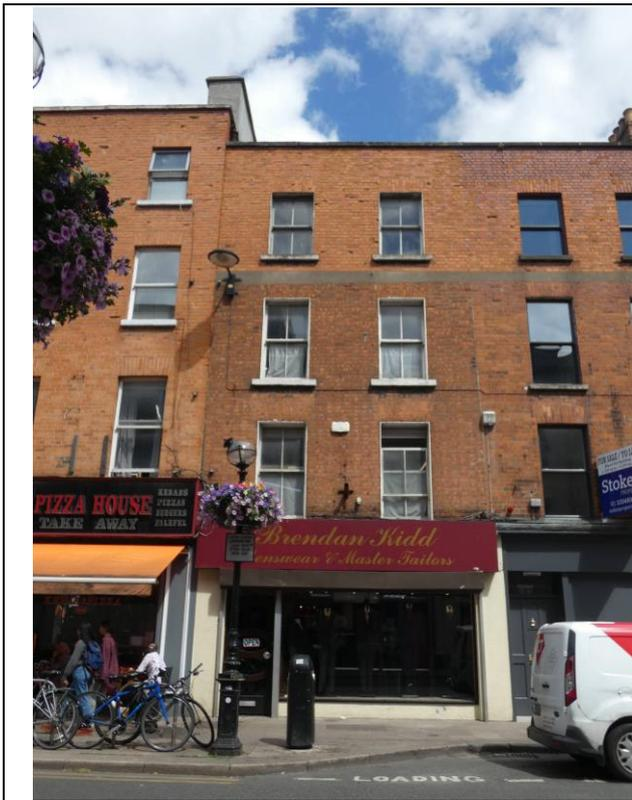
Fig. 3: Front (west) elevation. Note the re-faced brickwork to upper level.
