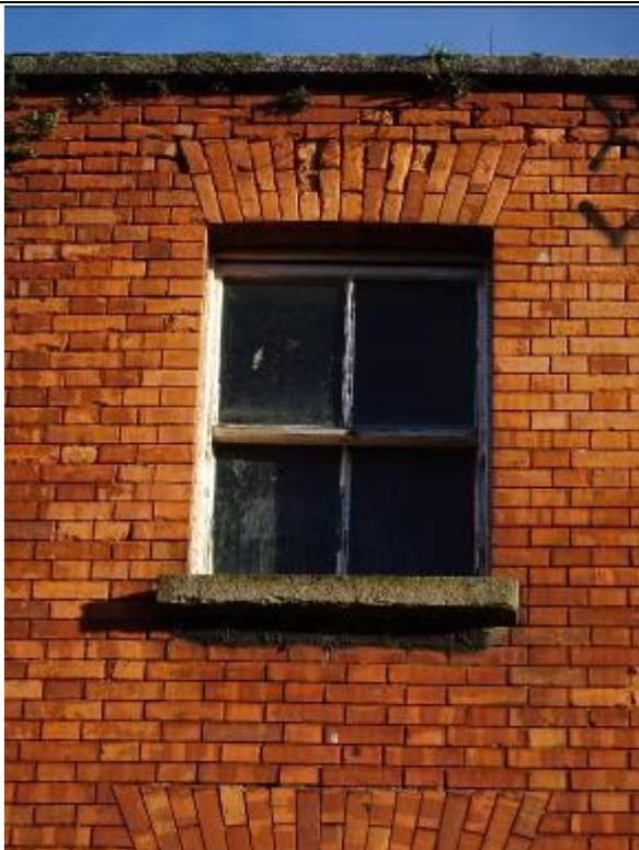
Fig.5: Detail of third floor window opening with granite cill and two-over-two timber sash window. Note the machine made brick to elevations laid in Flemish bond.
