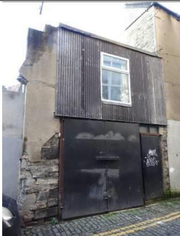
Fig.6: Two-storey mews building/warehouse fronting onto Jervis Lane Upper (known as both 56A Capel Street and 56 Jervis Lane Upper). Note the exposed sections of coursed calp limestone and brick masonry to lower level.
