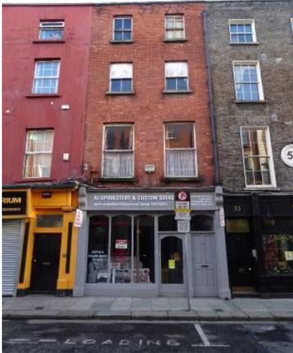
Fig.3: Principal/west elevation. Note the machine made red brick façade reflecting a re-facing of the early 18<sup>th</sup> century building c.1900.
